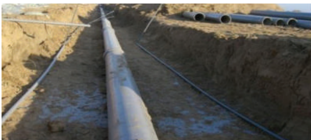
© North Korea Pyongyang Municipal Highway drainage project
