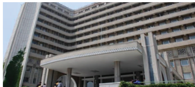
© ICRC North Korea hospital renovation and expansion
